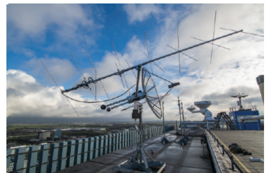
VHF/UHF/S-band 2m Ground Station
